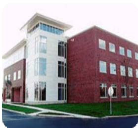
The Lupurt Building
